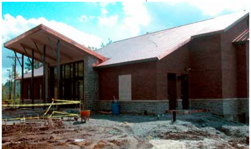
The new City Hall is quickly taking shape.
